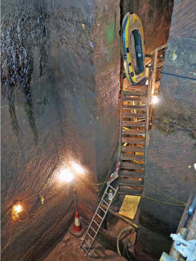
The temporary scaffolding staircase down into the reservoir, with the rubber boat required when it flooded not long before SubBrit's visit! Photo Clive Penfold
